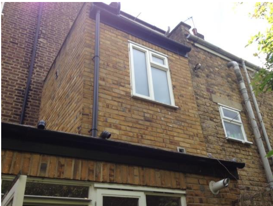
View of rear of No. 9 Patshull Road
