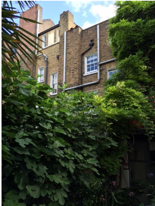
Photo 2: View towards no. 159
