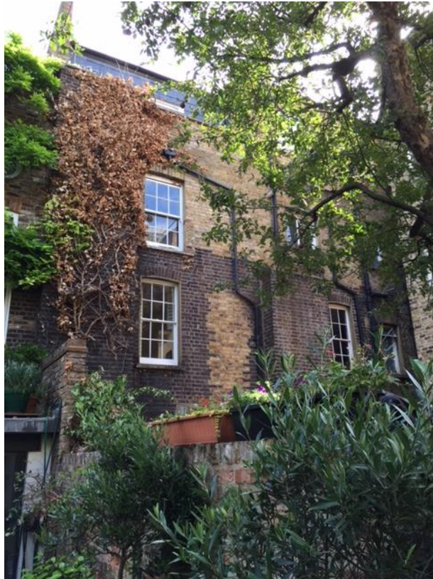
Photo 3: View towards no 155
