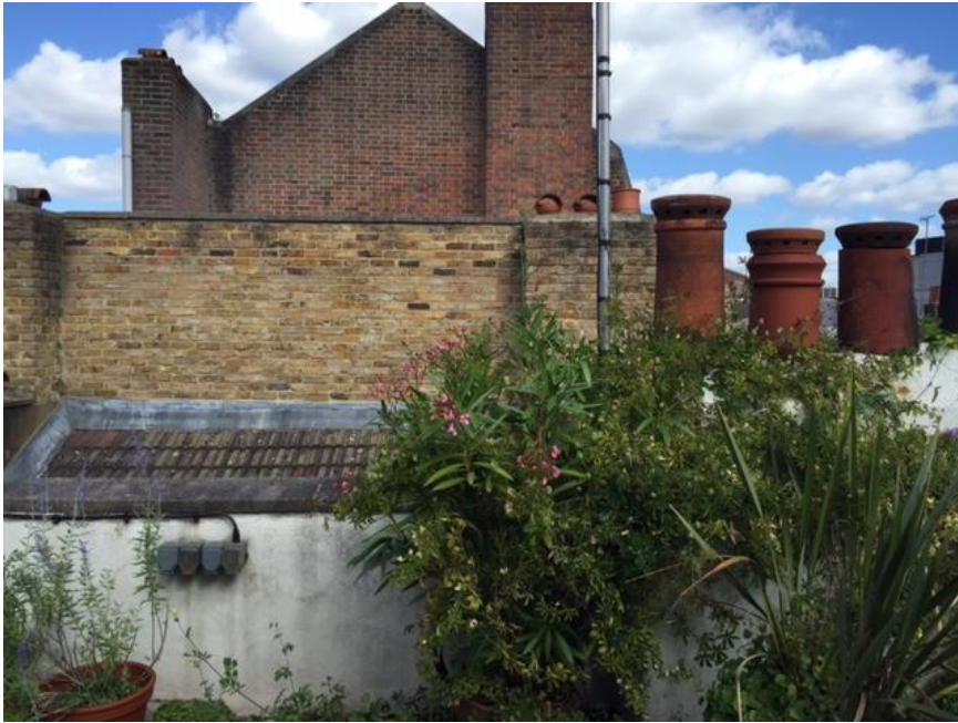
Photo 7: View of neighbouring roof at no. 159
