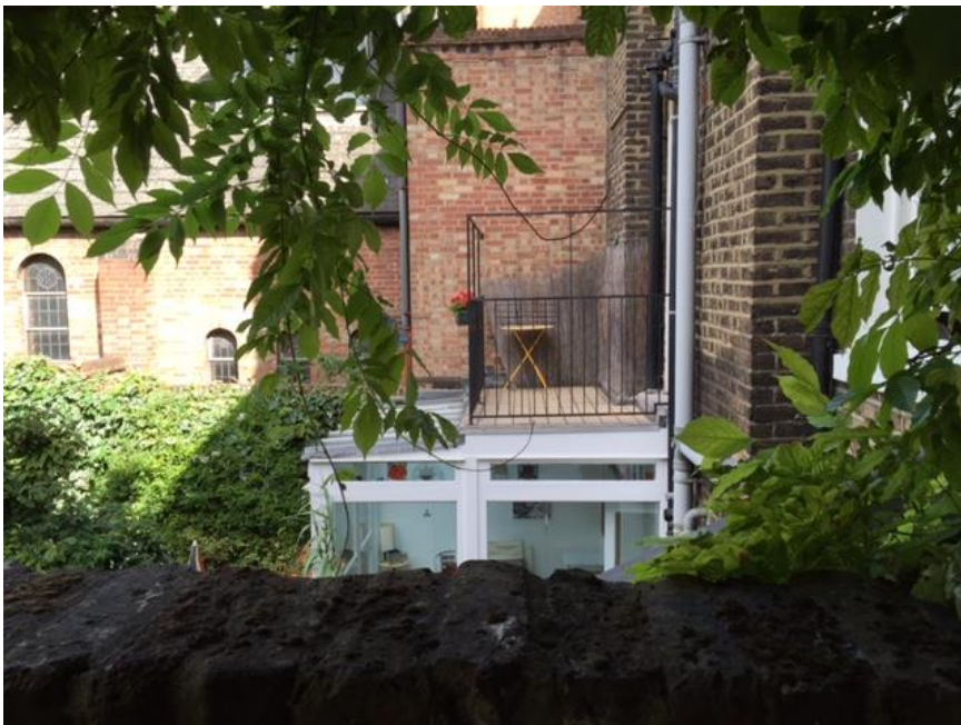
Photo 4: View from the first floor balcony showing railings at no.161
