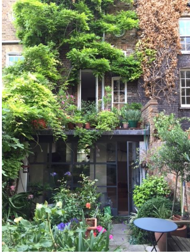
Photo 1: Rear elevation of the host building
