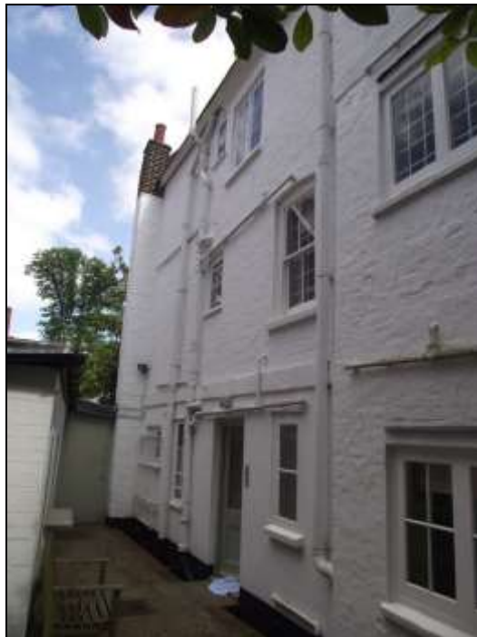
Plate 5 - North elevation with painted brick work and window insertions
