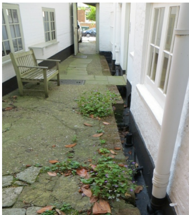
Existing channel next to rear wall where ground is to be lowered.
