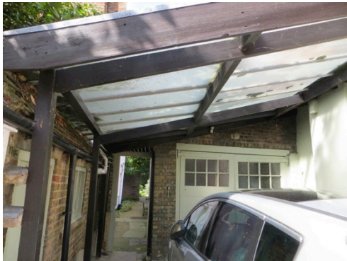
Existing timber and wired-glass car-port roof
