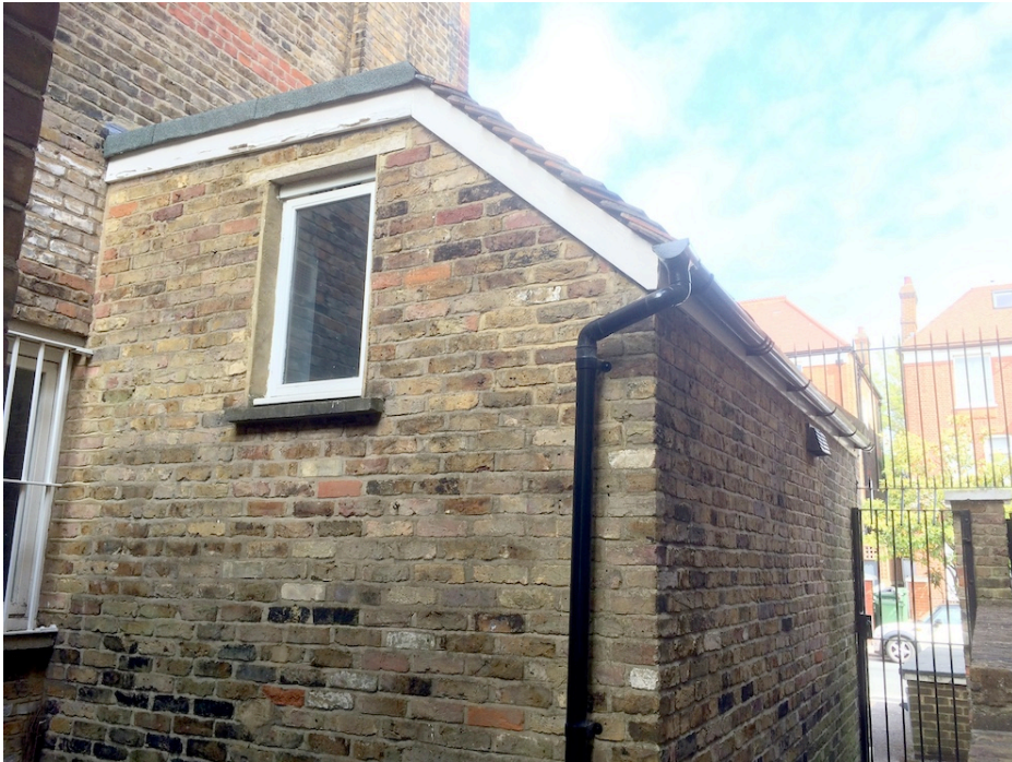
Rear internal elevation
