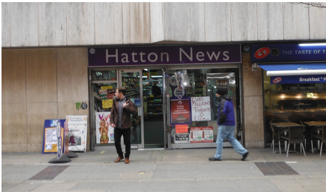
view 1 : existing A1 shop frontage
