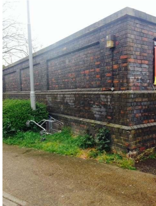
View of adjacent brick wall to railway ventilation shaft
