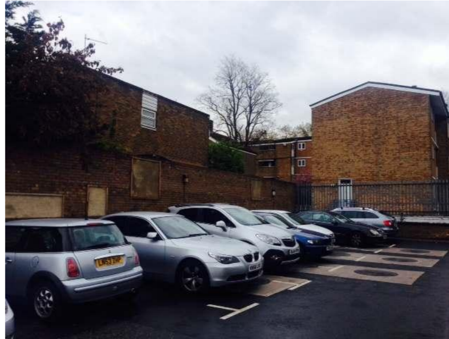
View to site from Tesco car park
