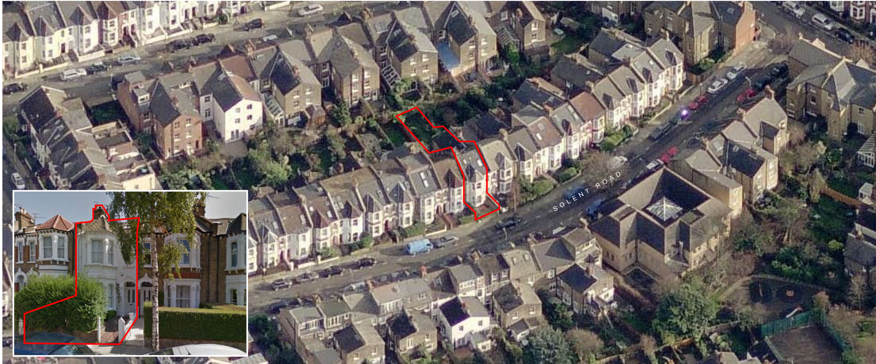
01. aerial view east and street elevation
