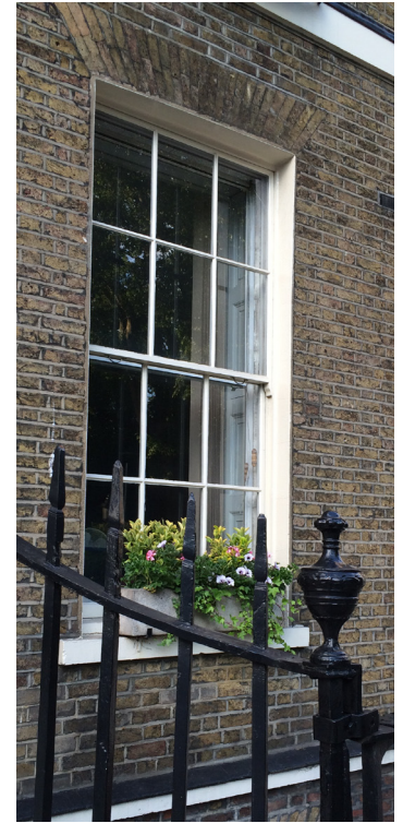
Secondary Glazing at No. 9
