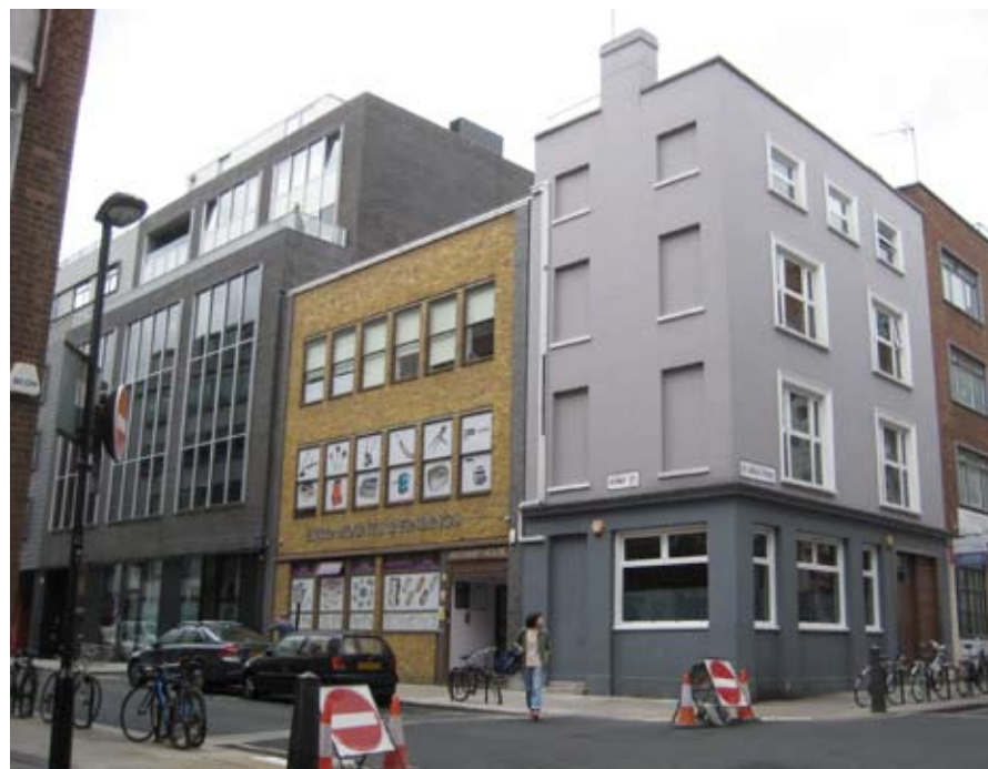
fig 02 08 junction of kirby street and st cross street
