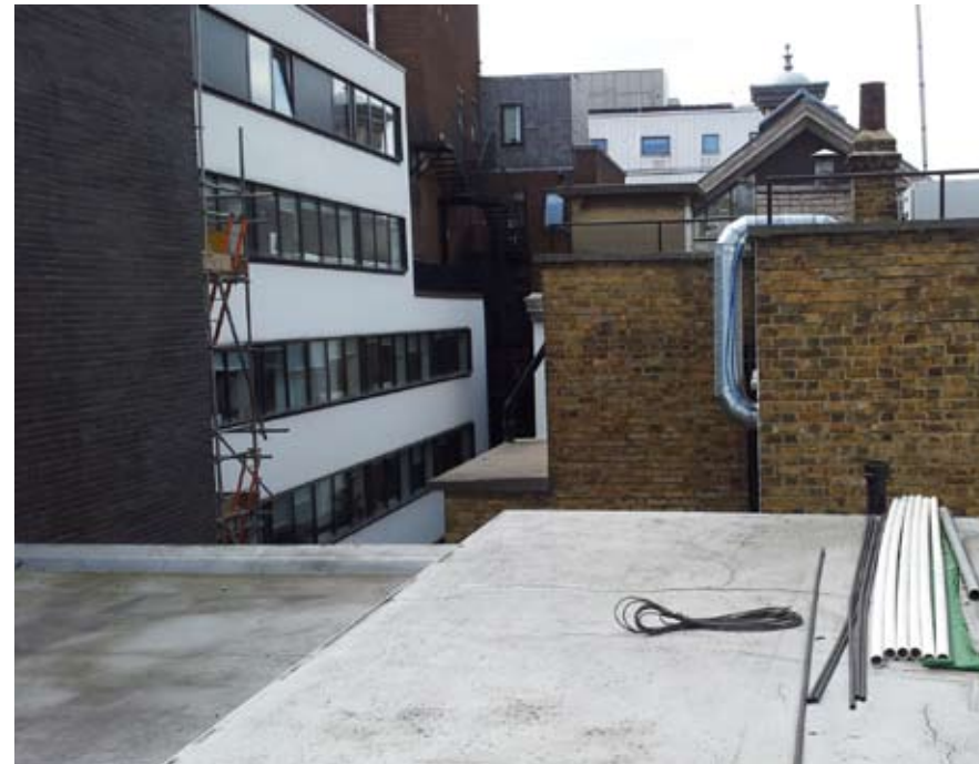
fig 02 12 view to rear of site from roof
