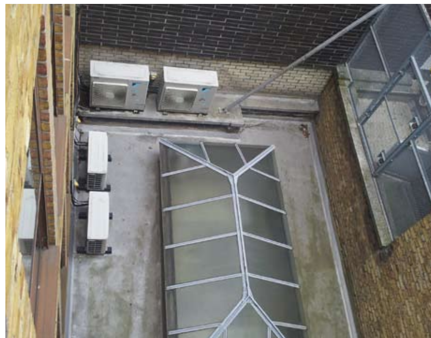
fig 02 14 view into light well from roof
