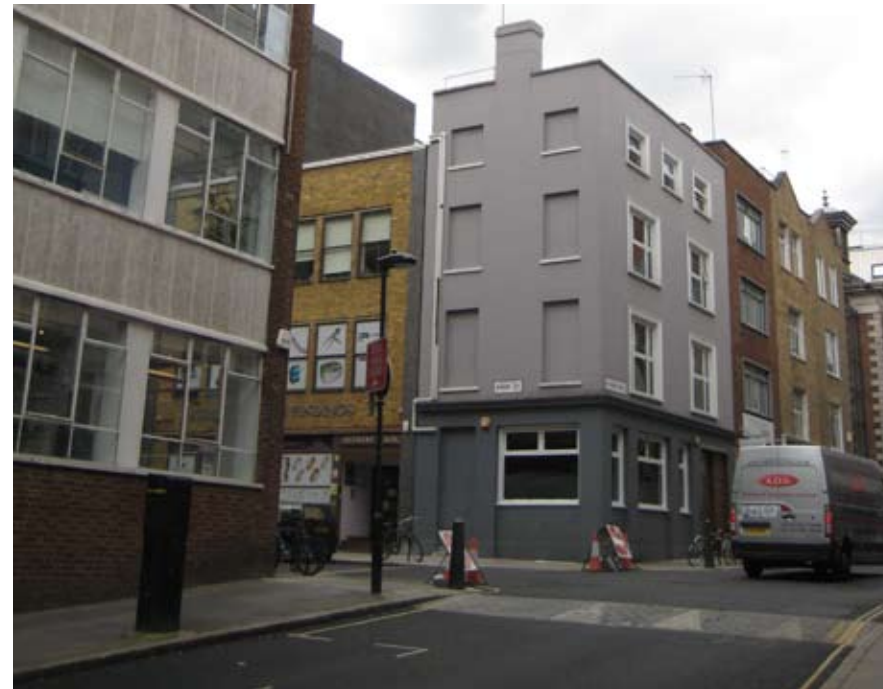
fig 04 14 junction of kirby street and st cross street
