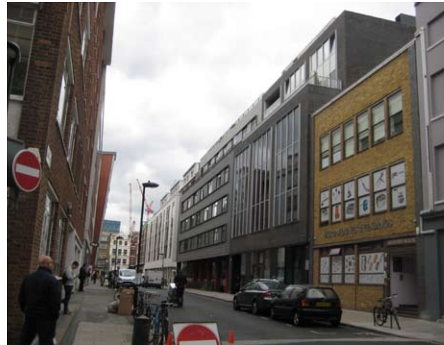
fig 02 07 kirby street from north with antwerp house in foreground
