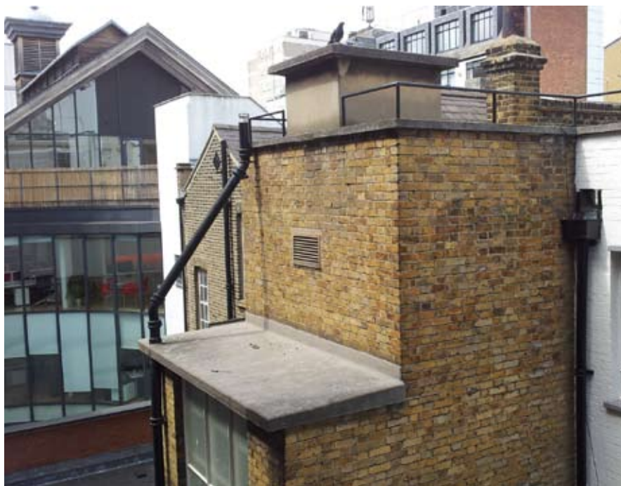
fig 02 13 view to rear of site from roof
