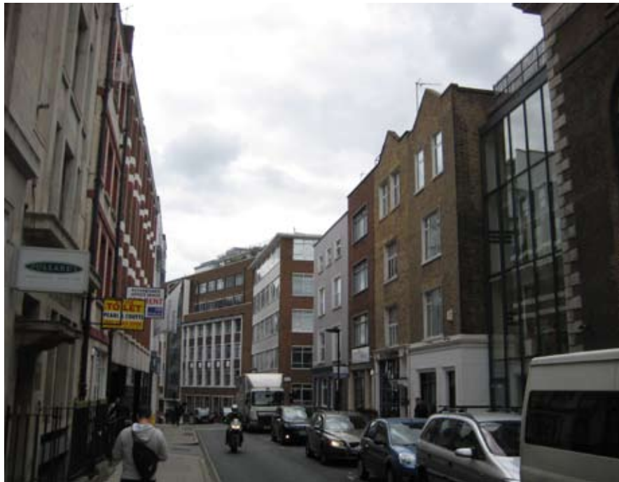
fig 04 13 buildings on st cross street
