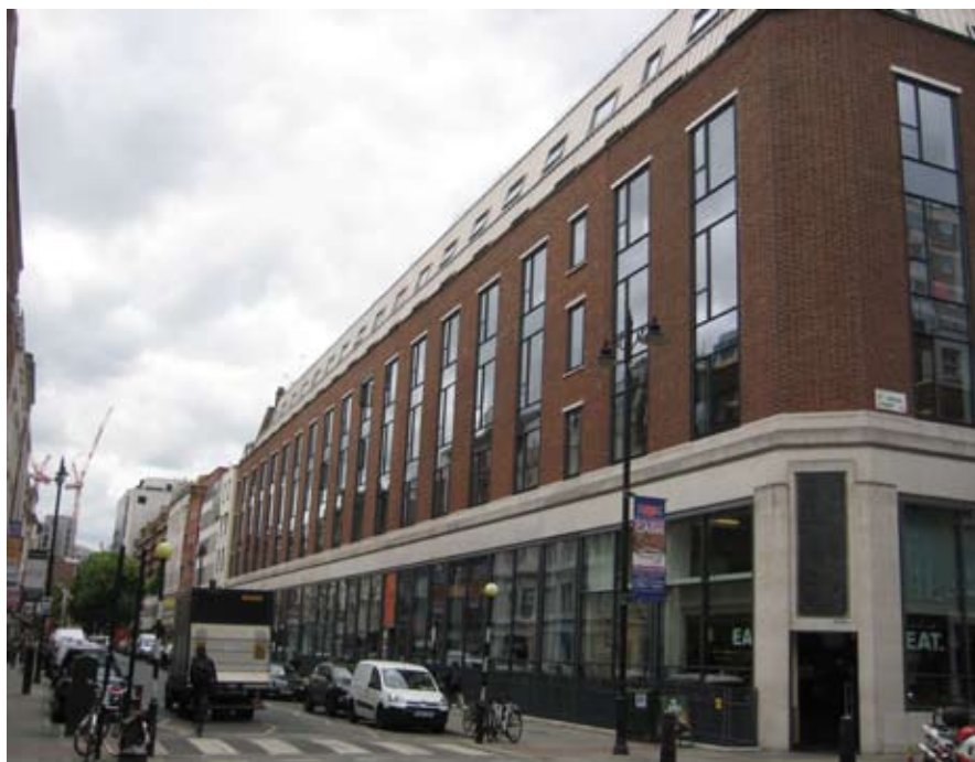
fig 04 11 typical traditional refurbished building in hatton garden
