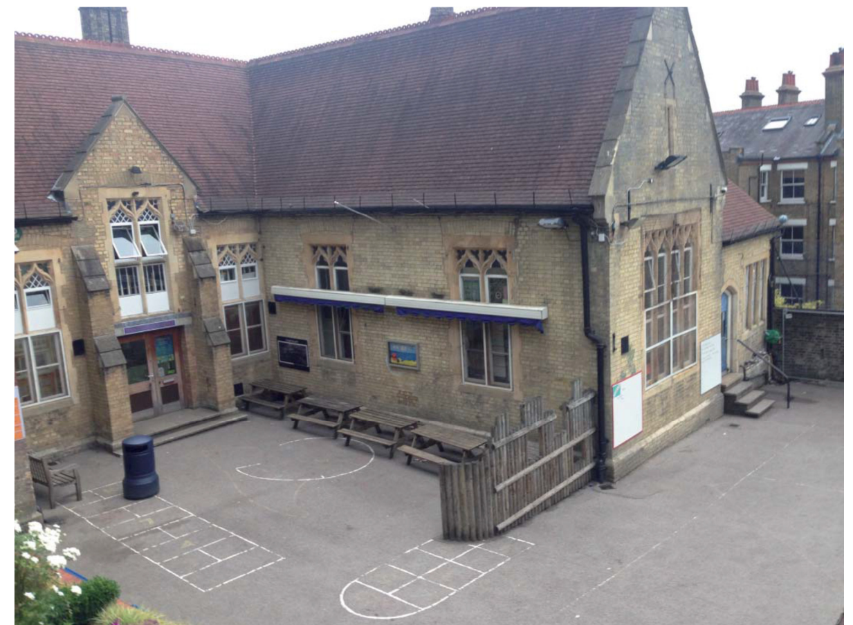
Fig 1 – Photograph of existing school building
