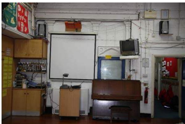
Gothic screen in Main Hall obscured by equipment
