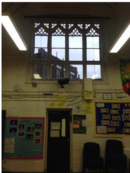
Tracery window in east wall of the Main Hall
