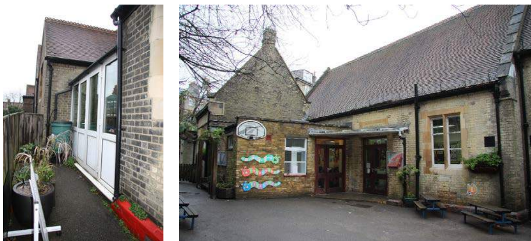
Left: Glazed Lobby, recently added between the nineteenth century girls' and infants' porches
