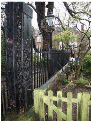
Railings along Christ Church Passage
