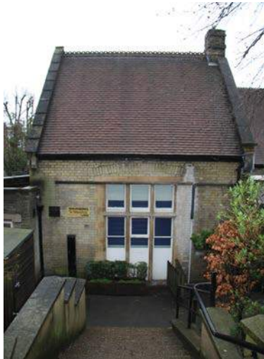
West Elevation of ICT Room (originally 1888 infant classroom).
