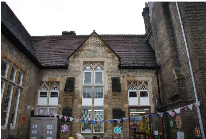
North Elevation of the school. A new door was inserted in place of windows in the 1990s and the glazing replaced some of the panes of glass when the mezzanine was constructed.
