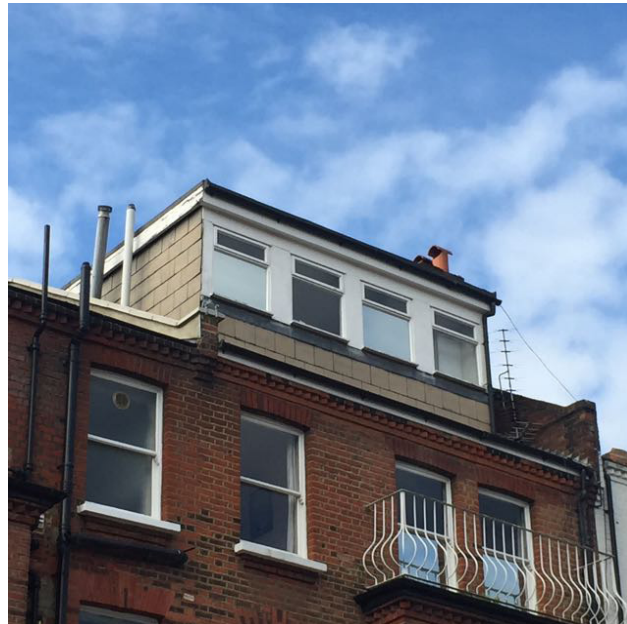
15 Carlingford Road. Oversized dormers with poor detailing
