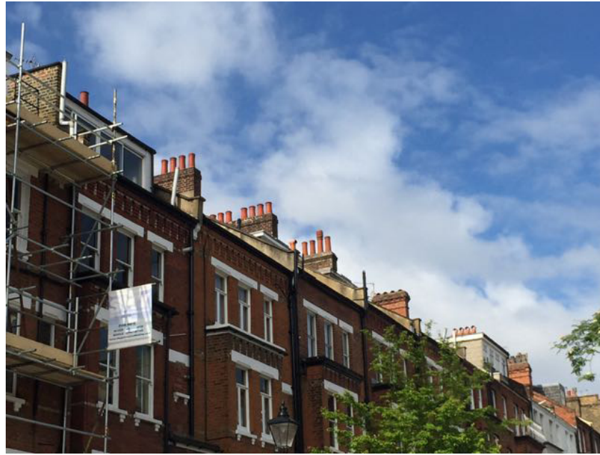
Carlingford Road - East Facing properties
