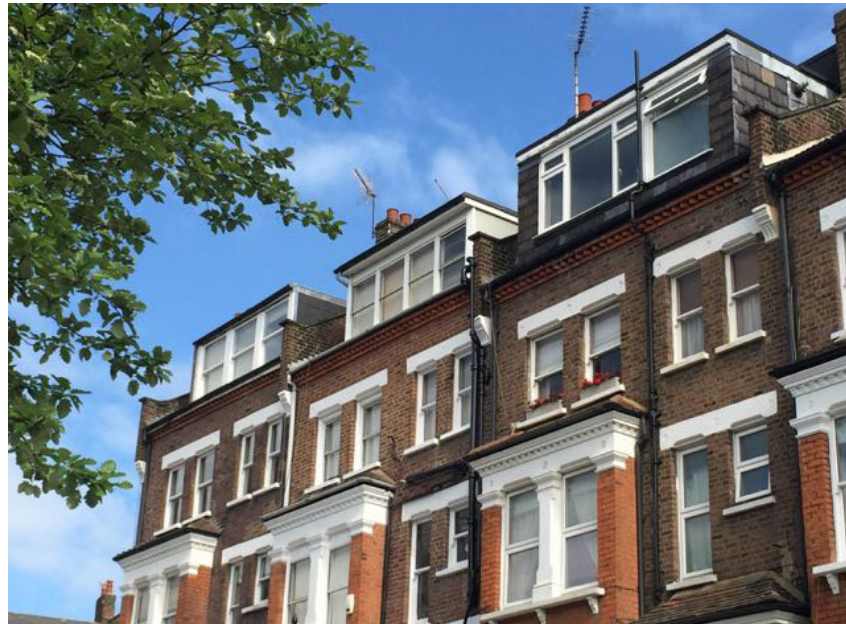
30,32,& 34 Carlingford. Oversized dormers project to the face of the facade
