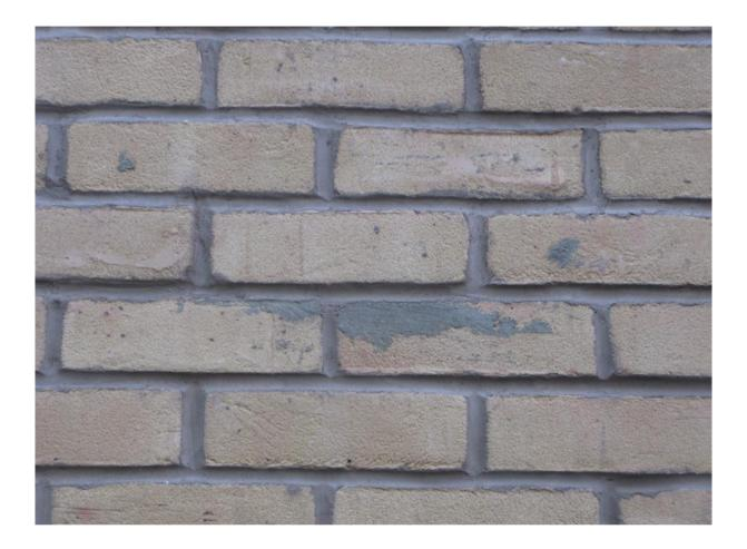
Unattractive design and poorly applied pointing work between bricks.
