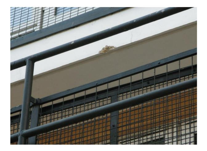
Detail of wall above front entrance. Not sure what this wall is made of or if done alongside recent works. Cracks in brickwork, top layer (of cladding?) coming away in parts, pointing missing in places. From a design point of view, it does not sit well with new plastering which has been carried out beyond entrance hall.
