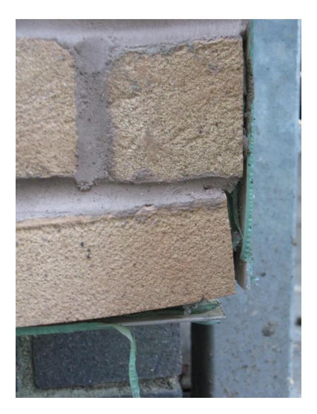
Uneven brick work halfway up side wall.
