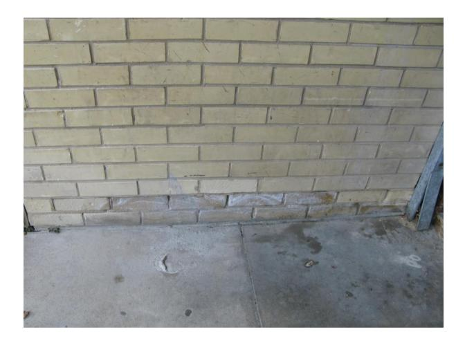
Details of area by entrance hall. Walls are stained. Unclear if these walls have been recently clad or if they have been done previously and not upgraded when recent cladding has been done.
