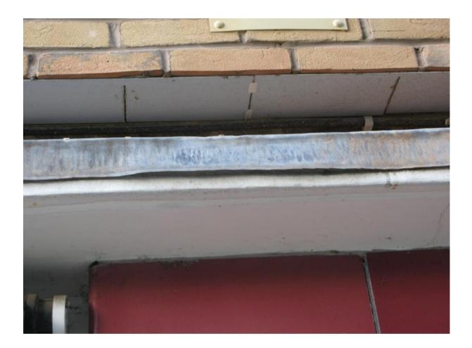
Unattractive design feature. Little thought has been given as to where the brick slips should end (as in what is the normal shape of a brick), or what the shape its cut into will look like once applied. The aluminium on the left does not appear to go right to the end of the slips.
