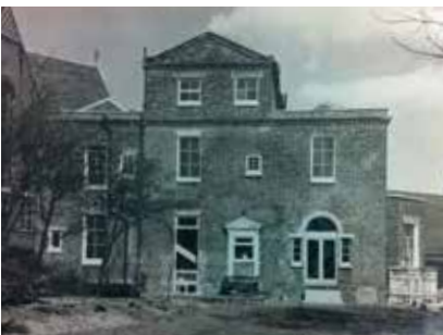
9. View of 11 Rosslyn Grove, east to west along entrance path, 1969. LMA
