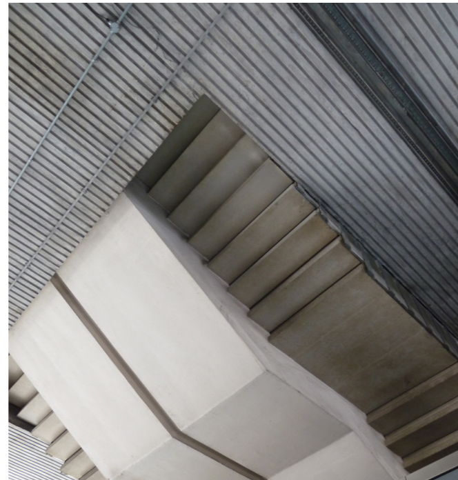
Underside of projecting stair
