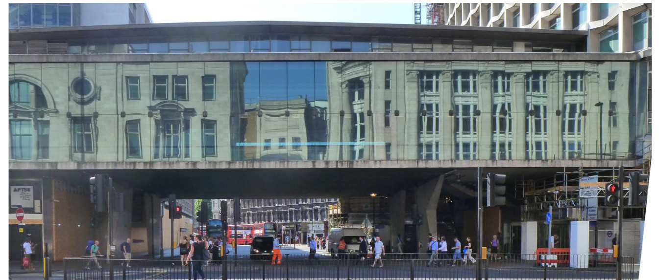
Top : Proposals for Infill Bottom: Centre Point link bridge prior to road closure
