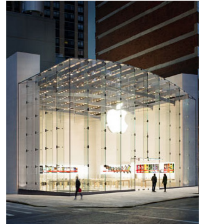
Apple Store, Upper West Side, New York Glass structural engineering by Eckersley O'Callaghan
