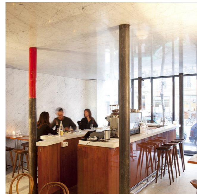
Le Dauphin, Paris. Uninterrupted soffit free of fixings.
