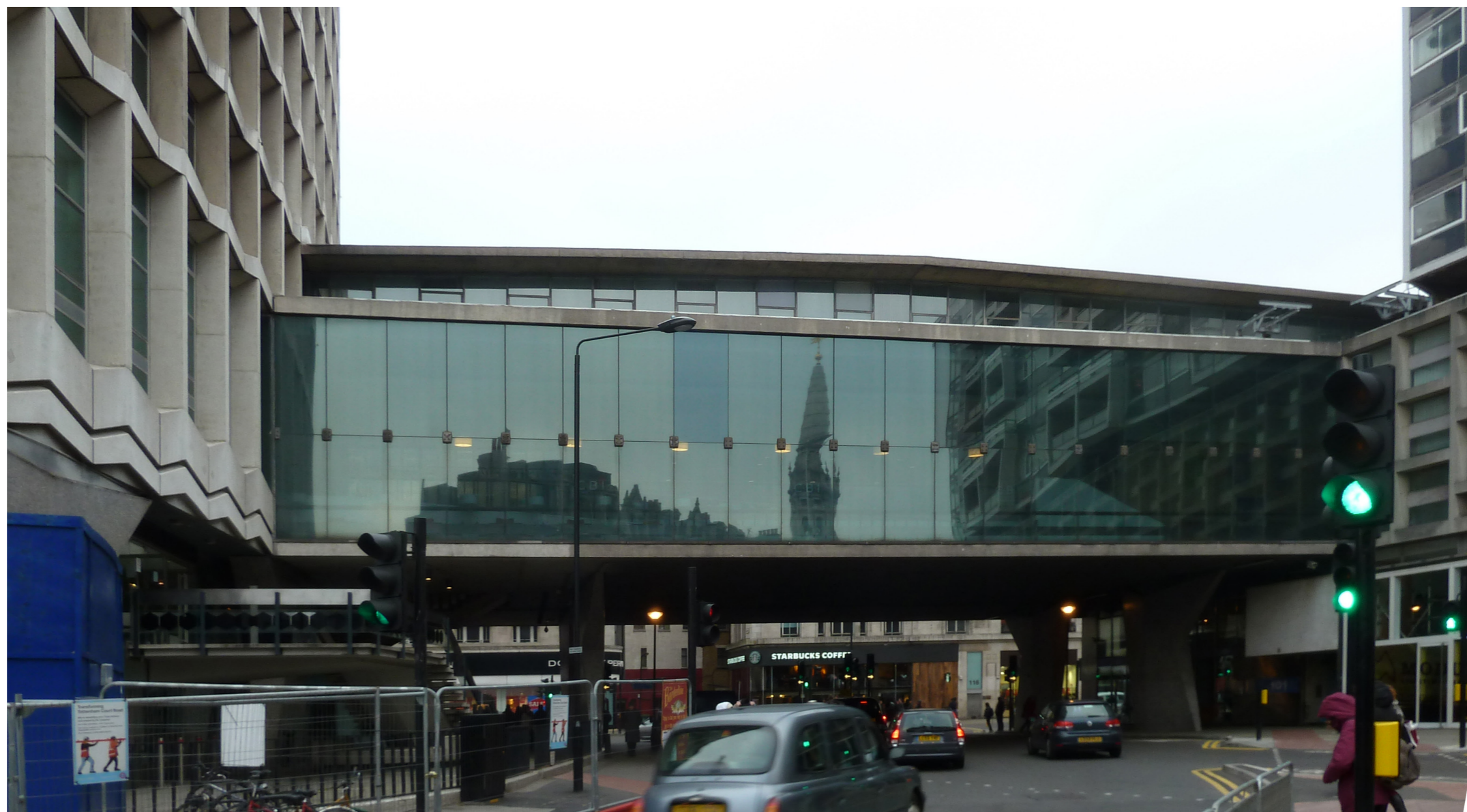
View from St. Giles Street to New Oxford Street: Existing
