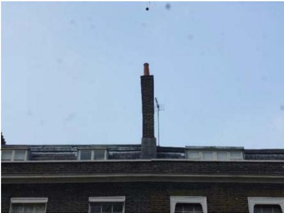
*Figure 1: Chimney between 21 & 22 Bedford Square to be rebuilt*
