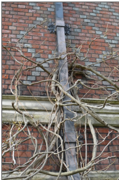
Twisted stems Obstructing pipe work
