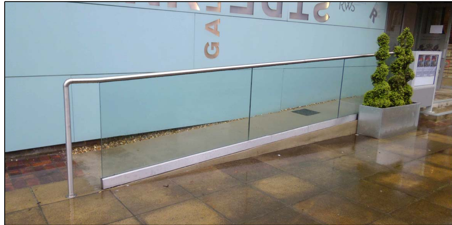
Typical stainless steel fixing / handrail detail to glass balustrade
