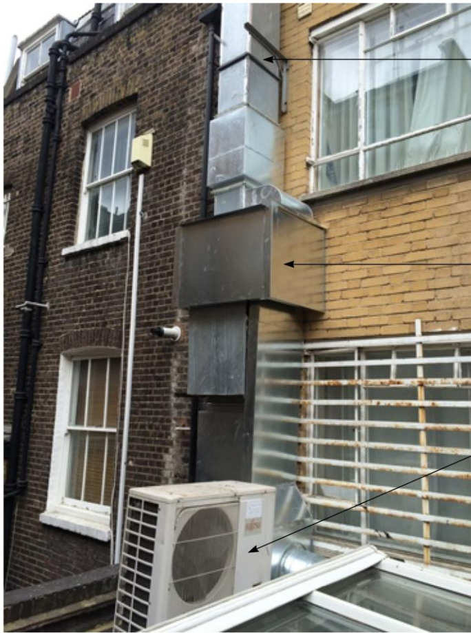
View of fan motor and duct and flue and also fujitsu air conditioning unit at rear, on flat roof.
