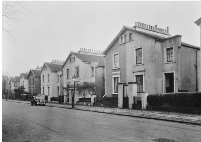
Figure 4 – 1-14, Provost Road, 1957 London Metropolitan Archives; SC_PHL_01_141_SL5474
