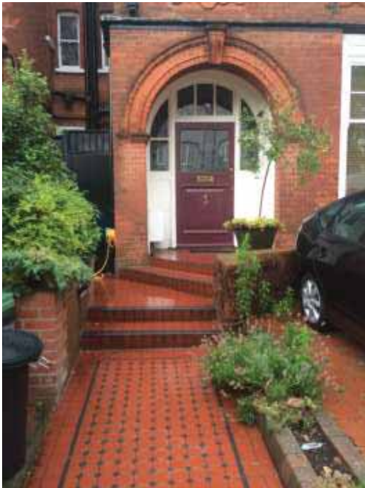
Photo No. 2: View of entrance porch.
