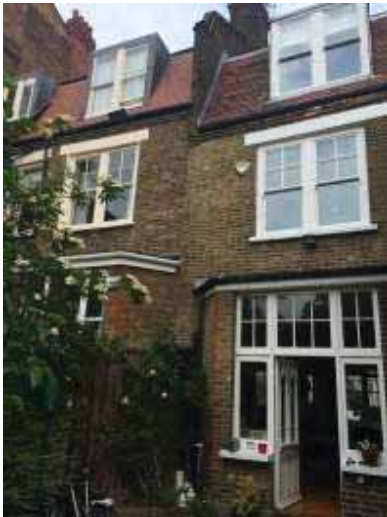
Photo No. 6: View of junction of nos 3 & 5 at the rear.
