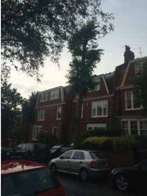
Photo No. 1: View of property from North-East. Note severely pollarded Elm tree in footpath.
