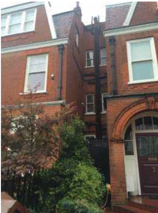
Photo No. 3: View of recessed attachment to no. 1. Note modern brickwork and pointing.
