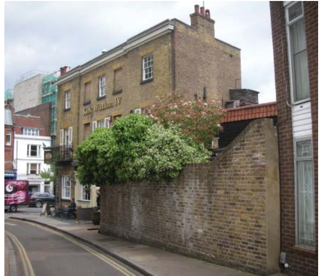
View of exterior of the garden wall from Perrin's Lane
