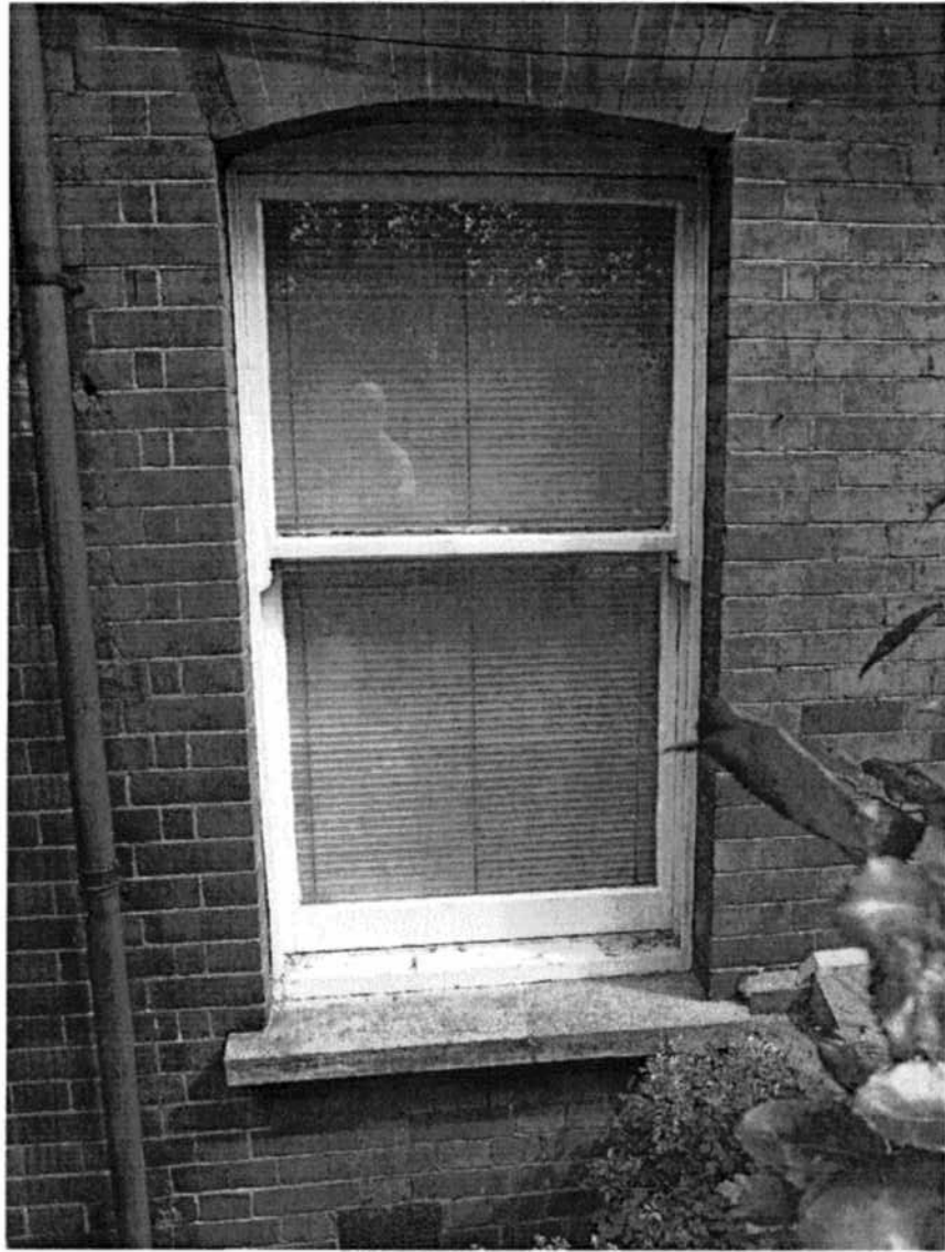
Window 5 on the front elevation of the property
