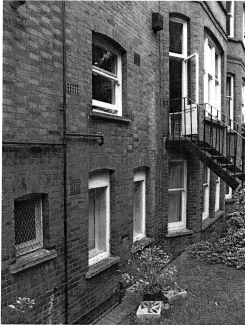
The rear elevation of the building
