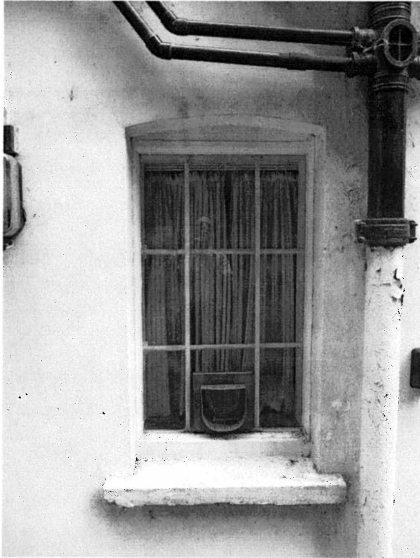
Window 7 on the side elevation of the property
