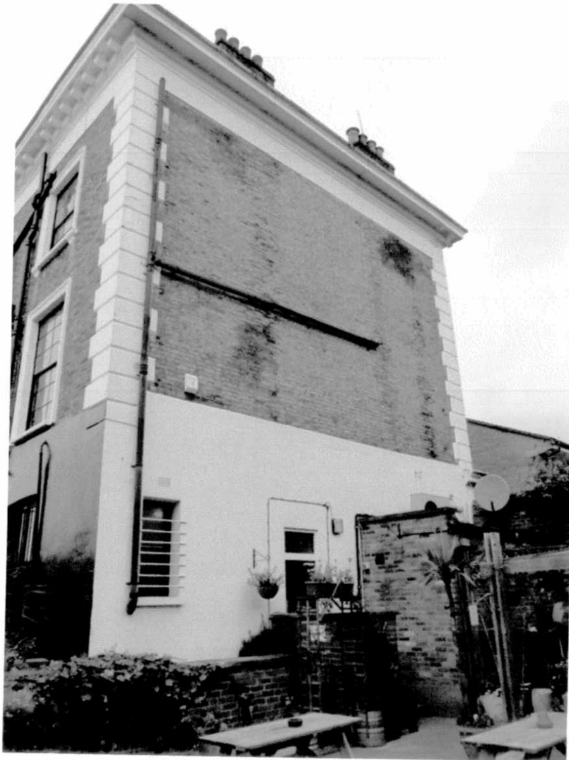
Figure 9. Eastern elevation facing the patio
