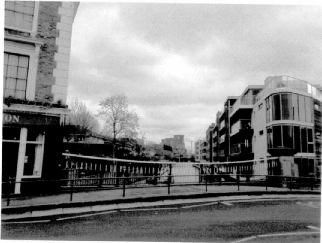
Figure 3. View east along the canal from Grays Inn Bridge
