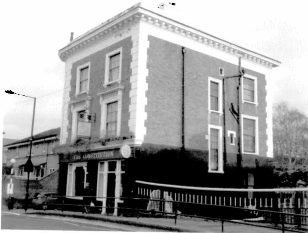
Figure 5. Southern elevation across the Bridge
