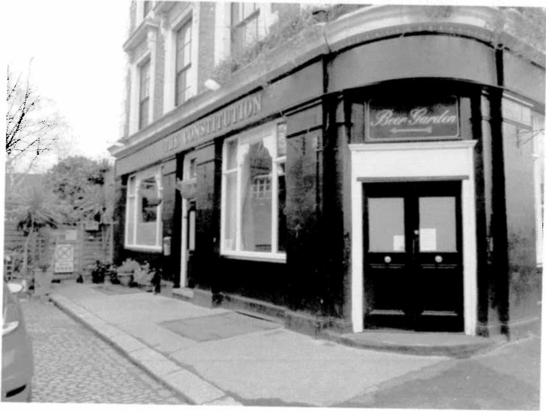
Figure 8. Northern elevation of the building
