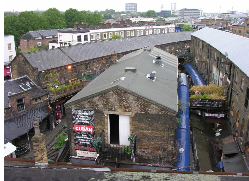
Figure 11 Current high level view of the Long Stable from the west showing the staircase canopy and link.
