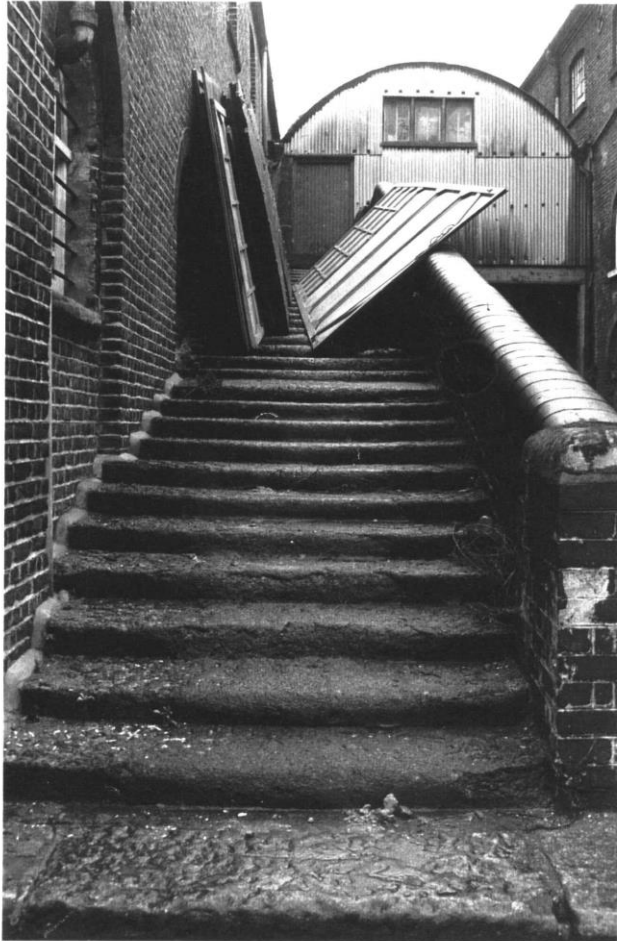
Figure 3 1975 photograph showing horse ramp to south side (now lost and replaced with a modern steel staircase).
