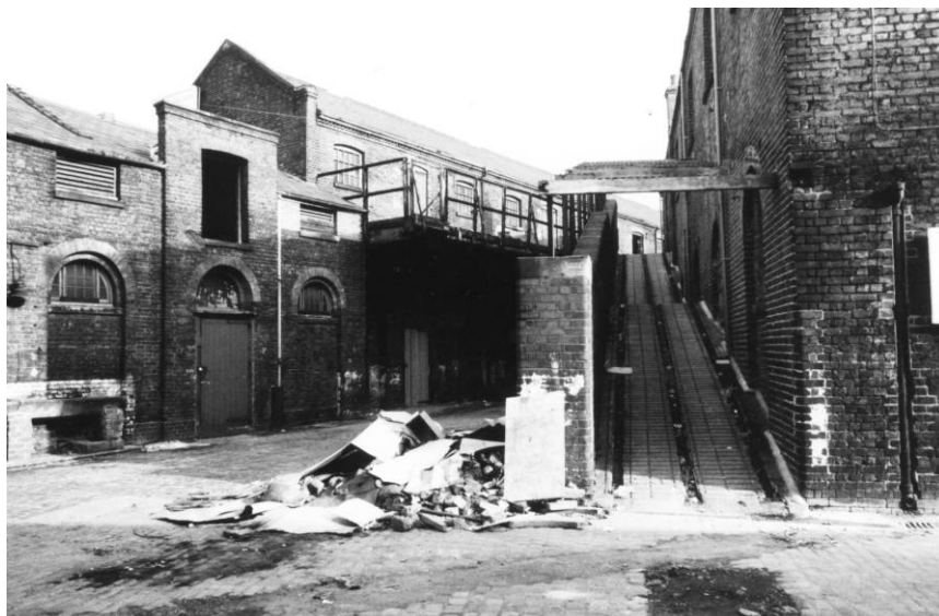
Figure 5 1975 photograph showing relationship between the Long Stable and the Chalk Farm Building viewed from the west. Note the canopy to the Long Stable horse ramp and the Chalk Farm Building walkway and balustrade.
