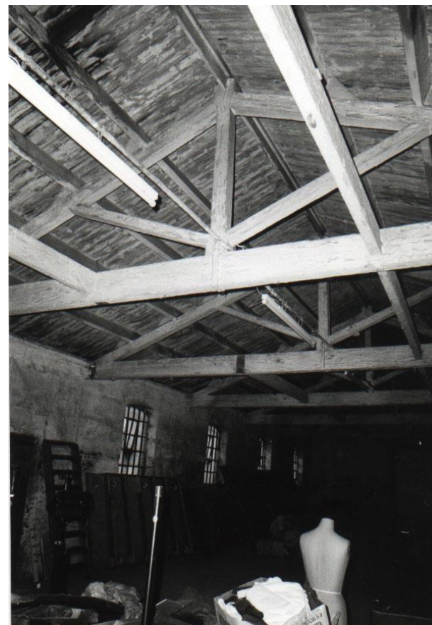
Figure 5 1975 photograph showing interior roof structure and sarking boards.
