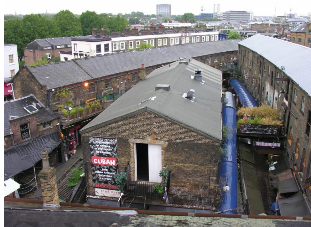
Figure 11 Current high level view of the Long Stable from the west. The roof fleche upstands still remain over the ridge.
