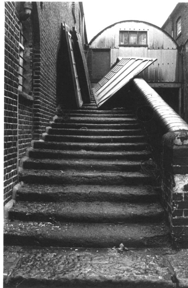
Figure 3 1975 photograph showing horse ramp to south side (now lost).
