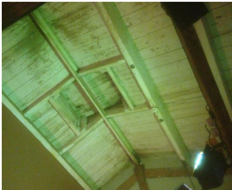
Figure 12 Internal view of roof structure showing remaining roof fleche upstand.
