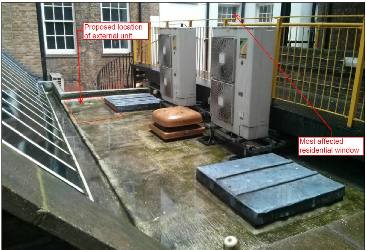
Figure 2.2: Rear External Courtyard – Proposed Plant Location
