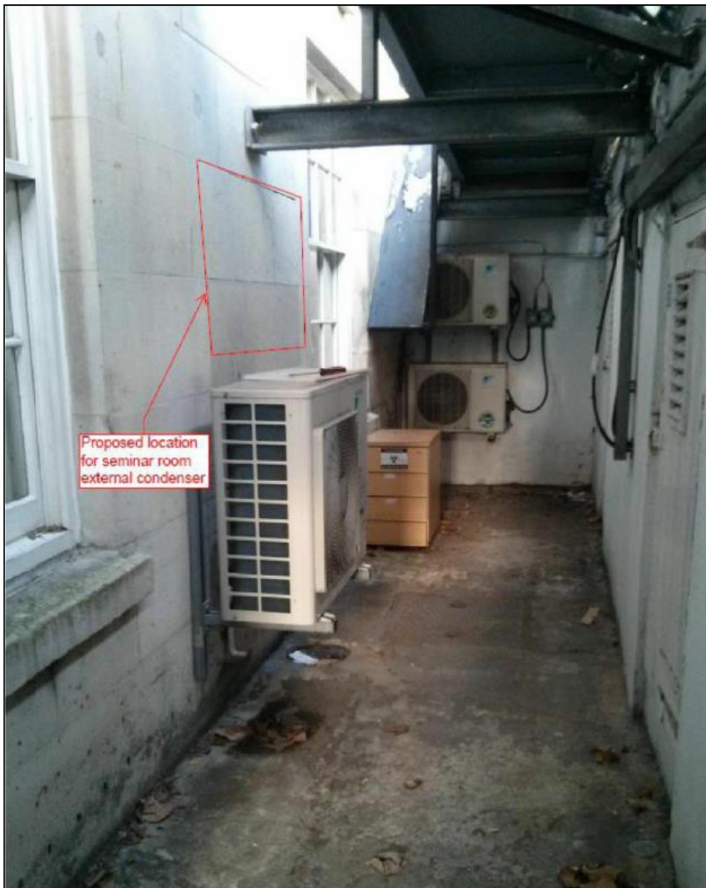
Figure 2.4: Front Lightwell – Proposed Plant Location
