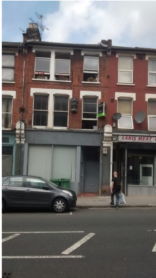
Figure 3 - Picture of the above-addressed property to Fortress Rd
