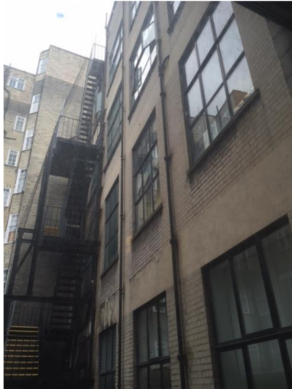
Photograph 3: Rear elevation of host property
