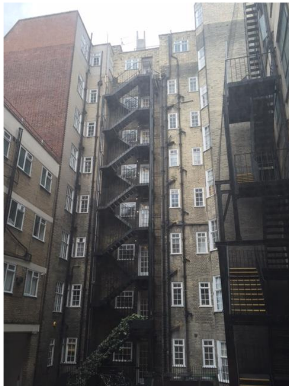
Photograph 4: Rear elevation of Queen Court to the north east
