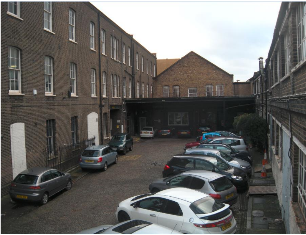
11. Internal Courtyard Area looking towards vacant principal building - 2012 when used for parking
