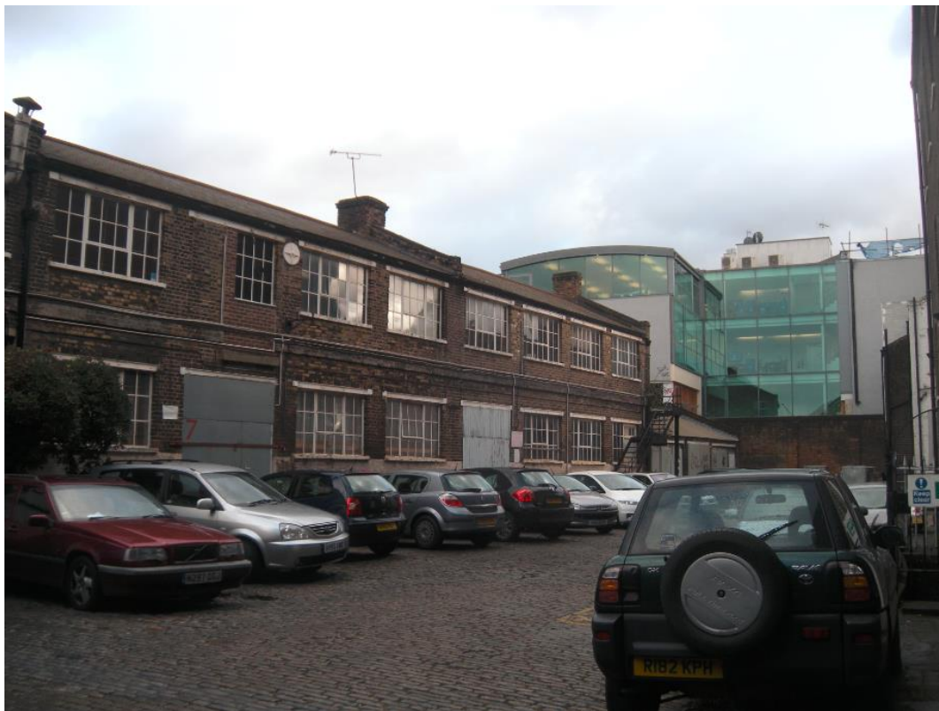
10. Internal Courtyard Area looking towards vacant light industrial building - 2012 when used for parking
