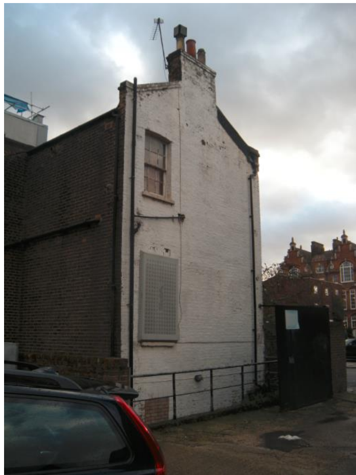
8. Side of Caretaker's House as viewed from access onto Gloucester Avenue
