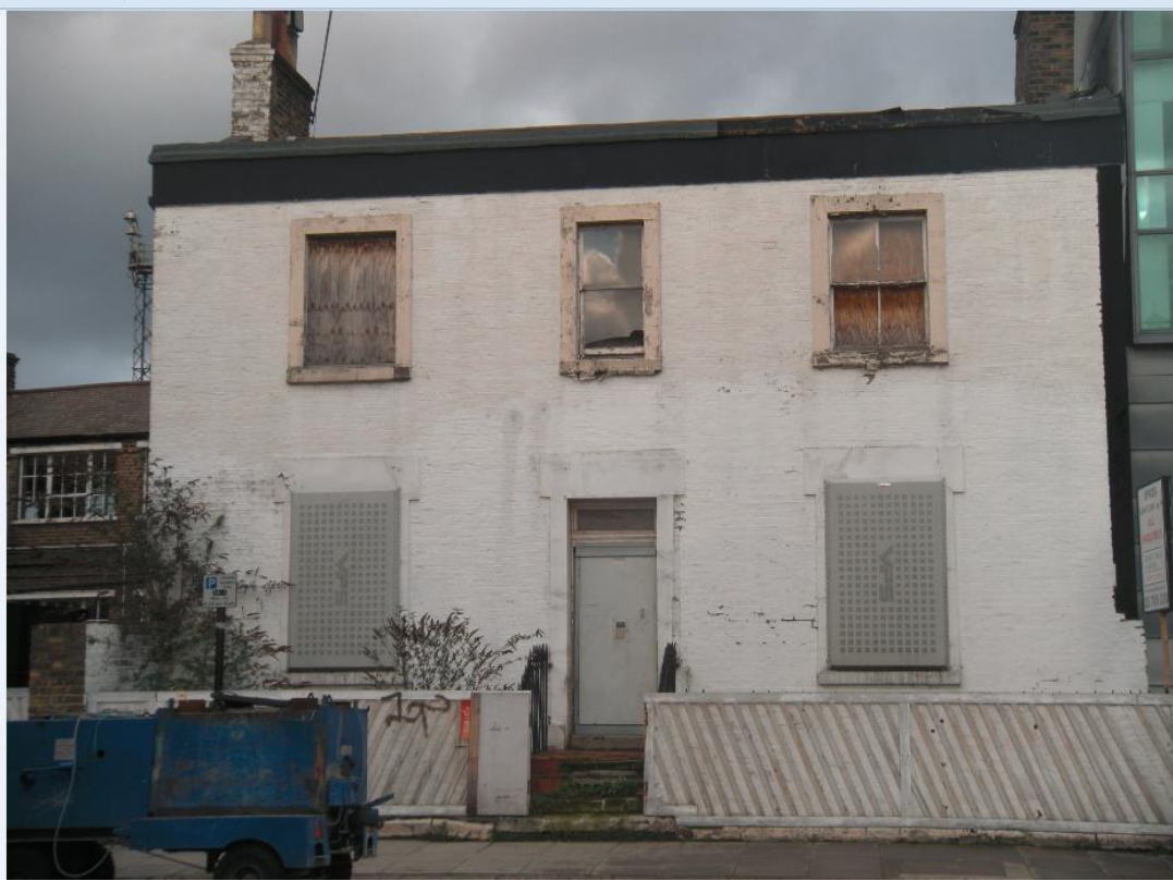
7. Caretaker's House as viewed from Gloucester Avenue
