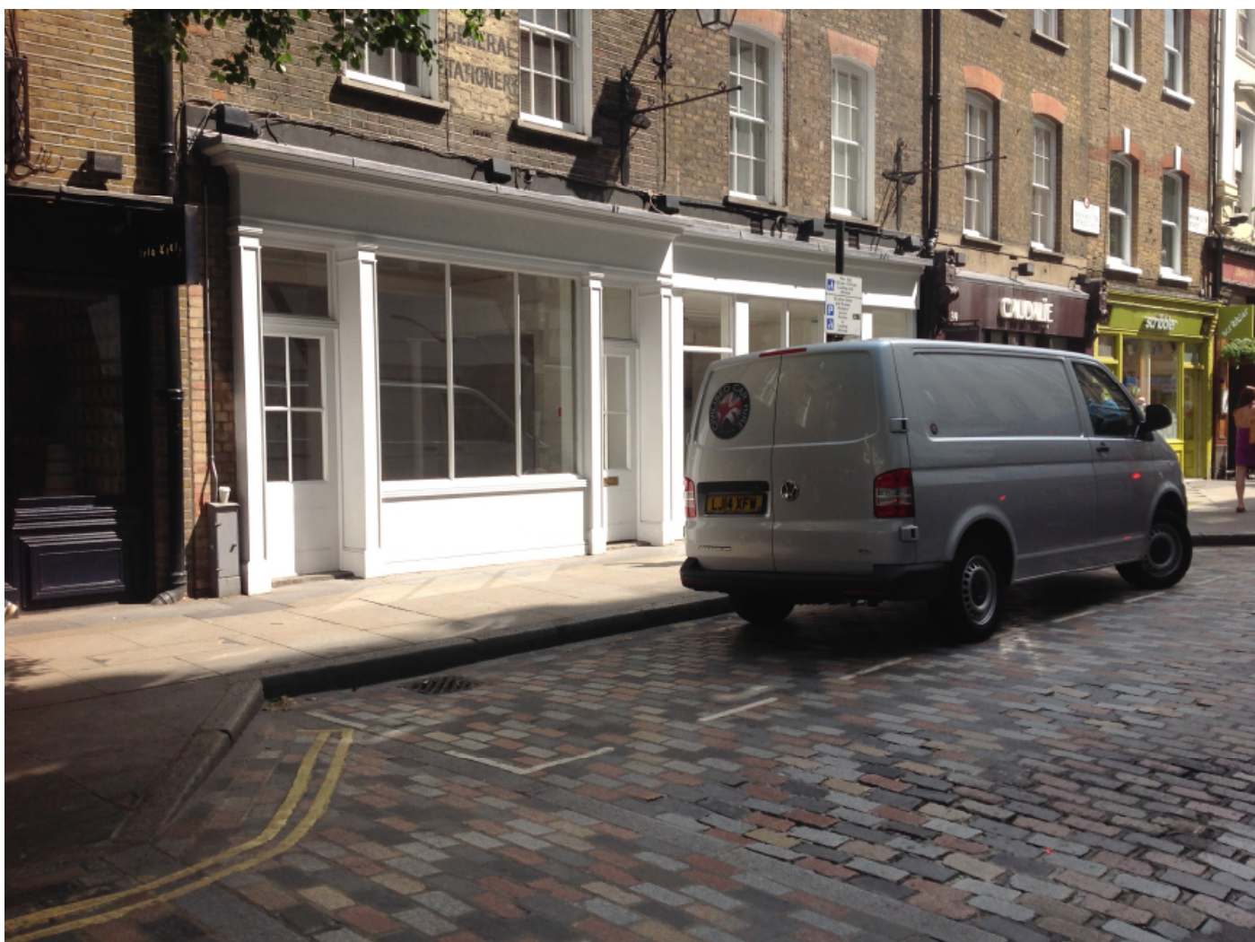
Photo 4: 35 -37 Monmouth Street (37 partially obscured by van)
