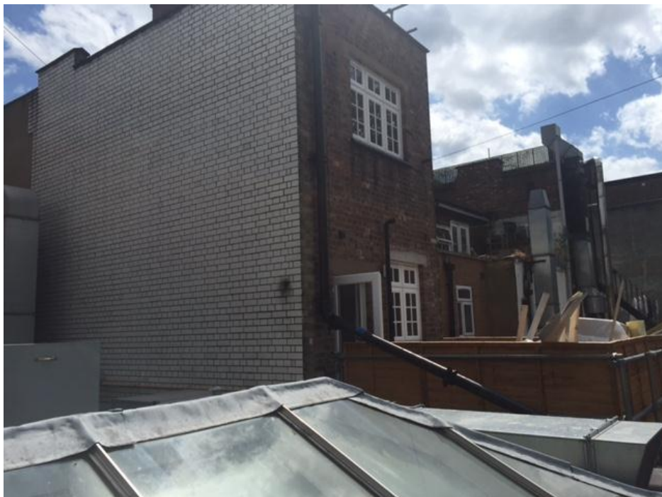
Photo 2: Rear projection of neighbouring property no.34
