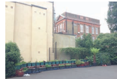
3 - Boundary to 10 Marsden St.
