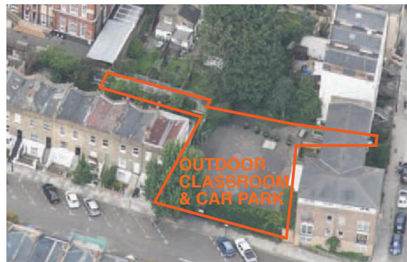
Aerial view of Outdoor Classroom & car park site
