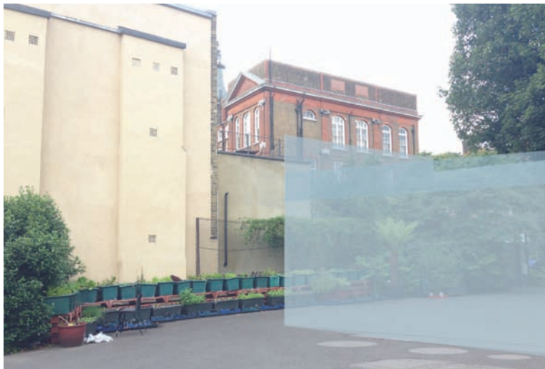
2 - View showing the proposed massing of the teaching kitchen in relation to the listed building (main school).
