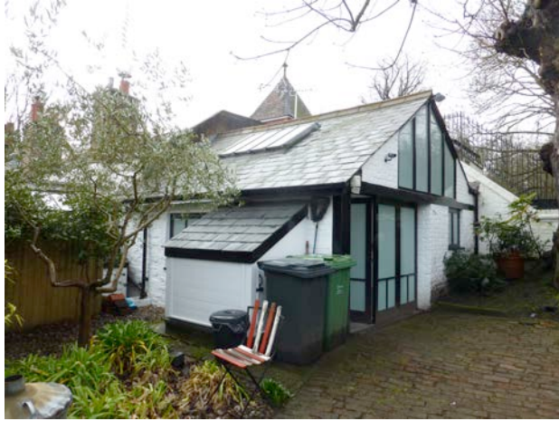
East elevation of separate garage/utility building
