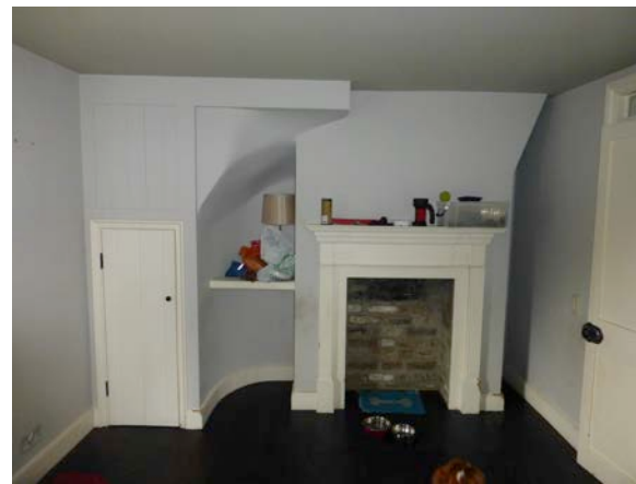
Original chimney breast with non-original fire surround and cupboard doors
