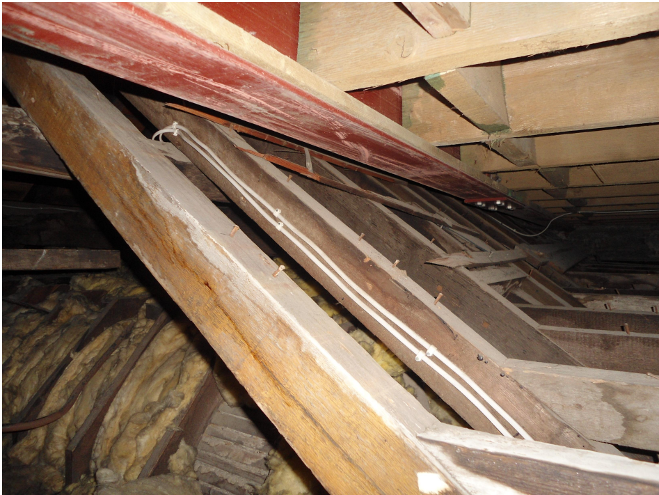
Figure 2 - Existing steel beam supports within loft space
