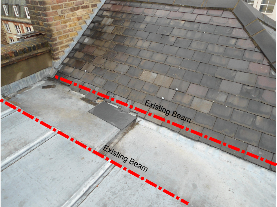
Figure 4 - Proposed Condenser Location in existing valley
