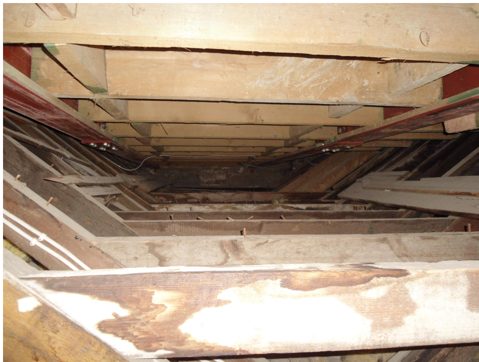
Figure 1 - Existing valley structure within loft space
