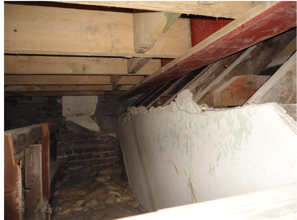
Figure 5 - Existing steel within loft space and original stud wall from 3rd floor level
