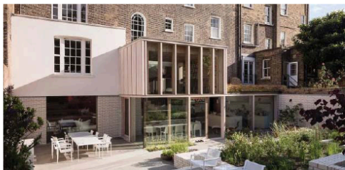
Example 1. East London house (David Mikhail Architects)
