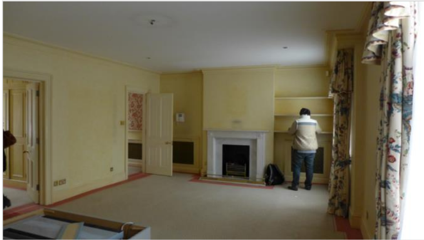
Figure 3.10: Previous condition of second floor front room
