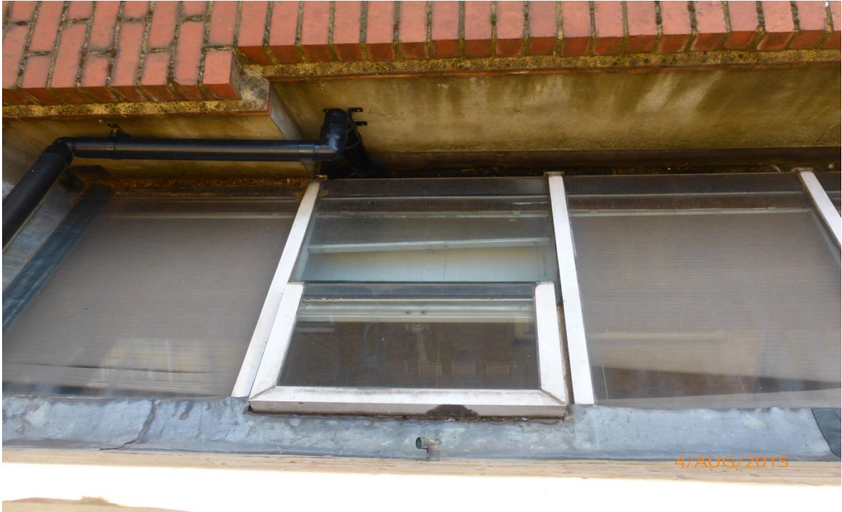
Photograph 1: the original skylight, ground floor
