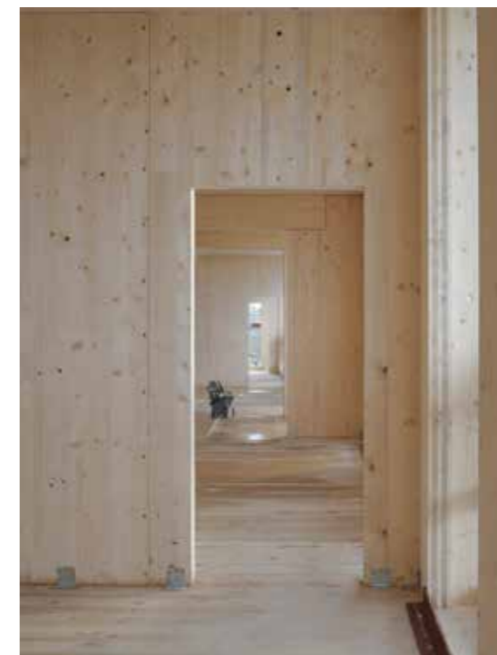
Precedent photographs of cross-laminated timber construction
