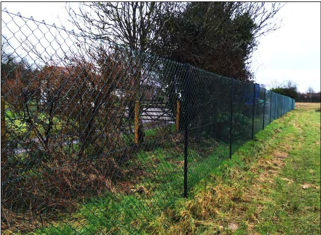
Chain-link on angle-iron uprights
