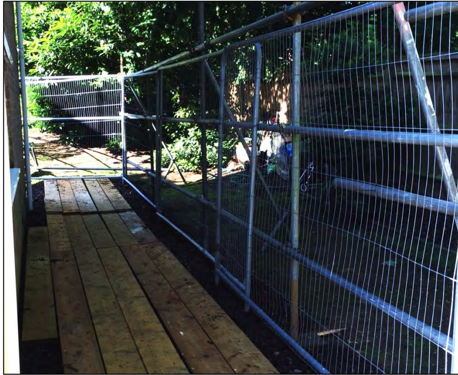
Scaffold board pedestrian ground protection
