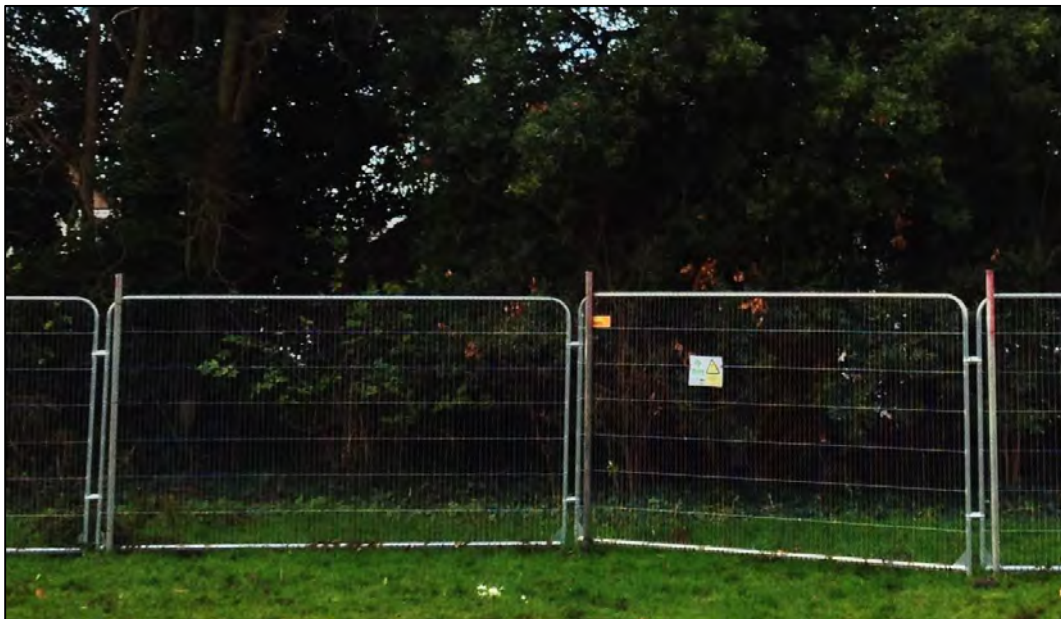
Weld-mesh panels on scaffold uprights
