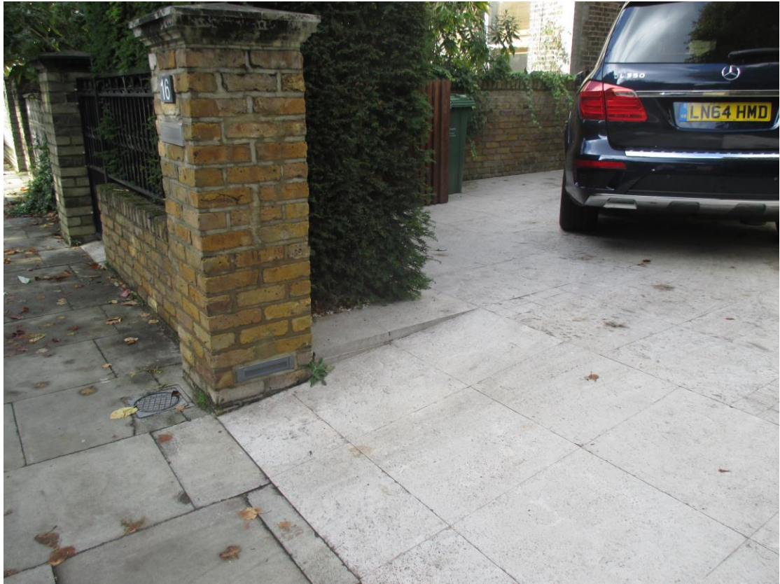
Photo 3- Forecourt Parking Left Hand Side (Existing)
