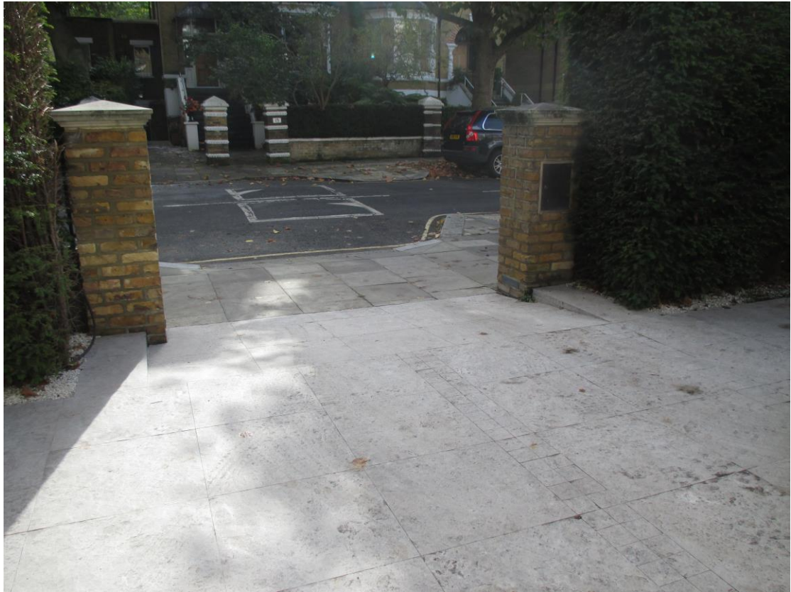
Photo 1- Existing Vehicle Crossover
