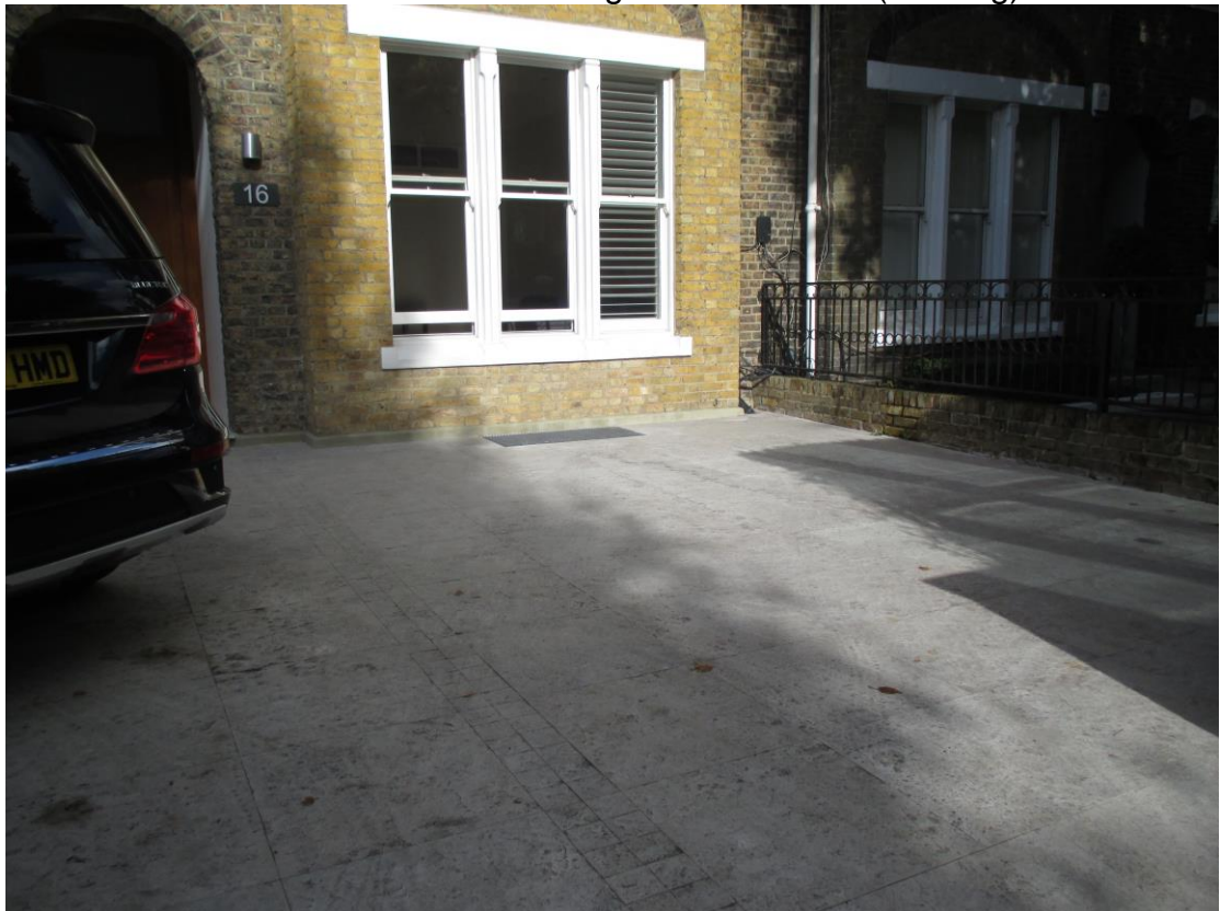
Photo 4- Forecourt Parking Right Hand Side (Existing)
