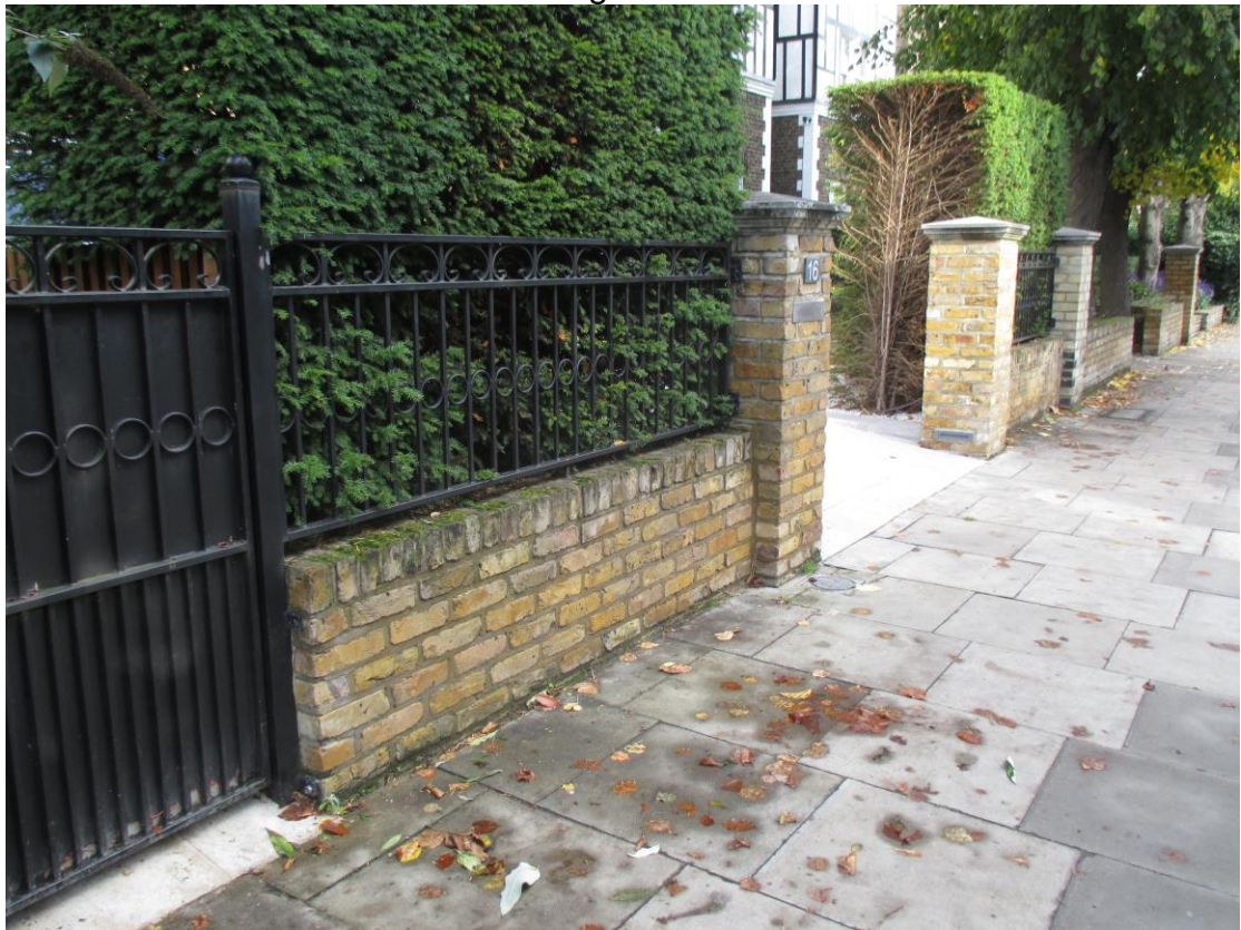
Photo 2- Front Boundary Treatment
