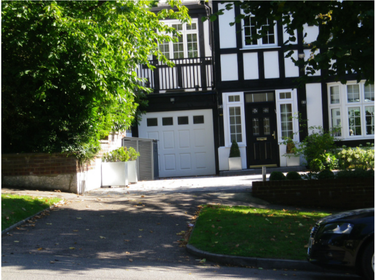
Similar design of neighbouring garage door
