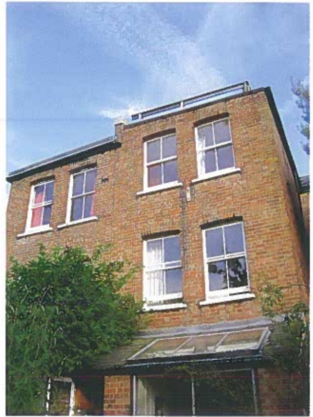
Existing ground floor lean-to and third floor terrace
