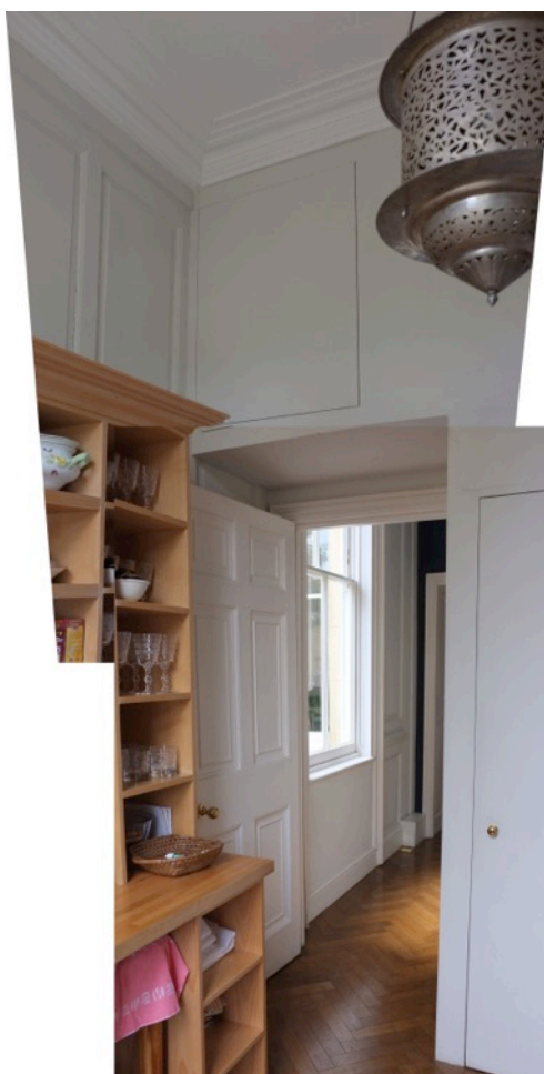
FG11: modern kitchen storage built as part of stair (to be removed; panelling and door retained)
